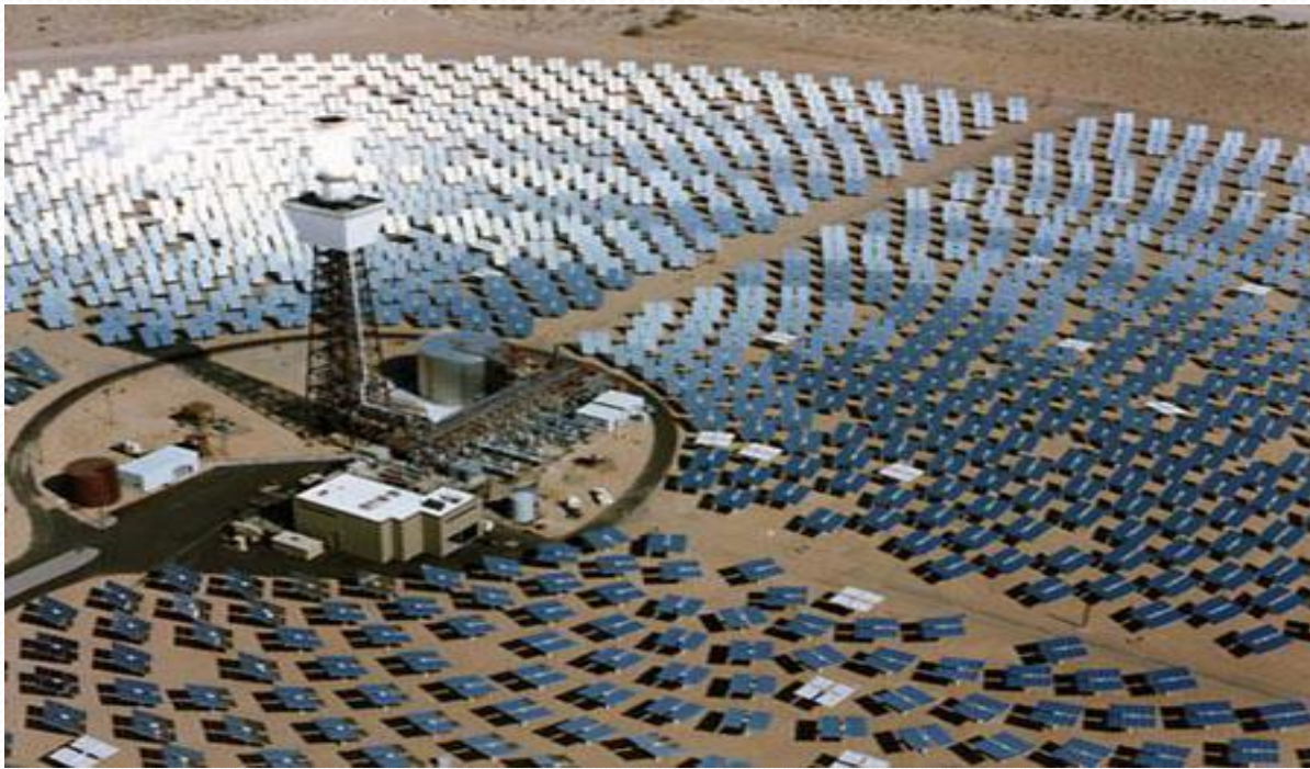
Power tower in Barstow, California.
